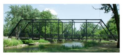
The simple answer is that triangles are stable. A triangle has three sides and, if these are fixed in length, there is only one configuration they can be in. There is no flexibility or freedom. On the other hand, a quadrilateral has more degrees of freedom. Without changing any of the lengths of the sides the shape can be deformed.
